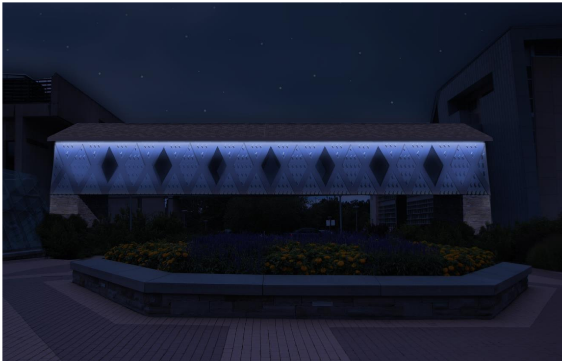
Figure 35: Exterior Lighting of the Bridge with Blue LED Light
