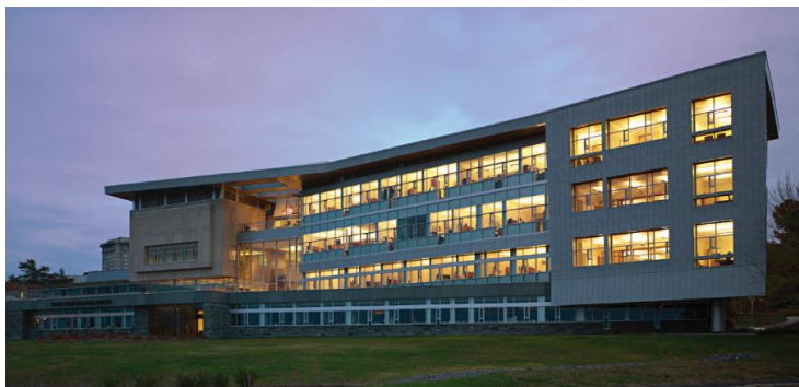
Figure 2: View from the North Showing Irregular Facade of the PRWC Photo provided courtesy of Holt Architects
