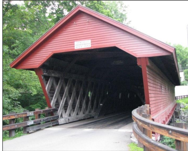
Figure 22: The Newfield Bridge | Photo taken 07-31-13
