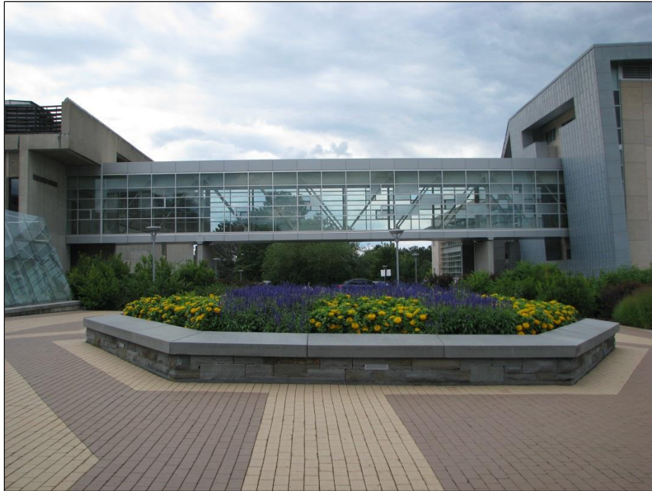
Figure 29: Existing Bridge Façade | Front View
