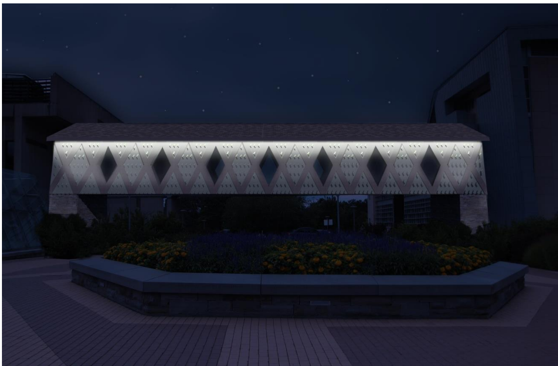
Figure 33: Exterior Lighting of the Bridge with Original White LED Light
